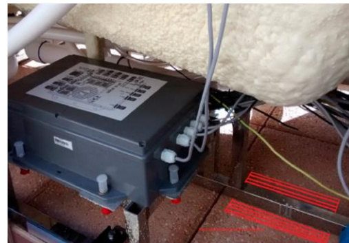
Floor level along support structure
